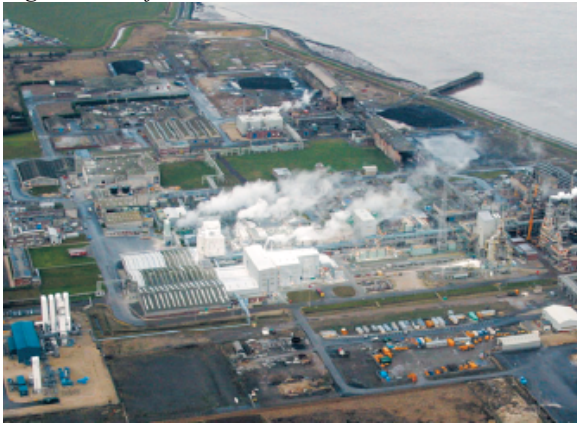
Fig 1: View of Site
